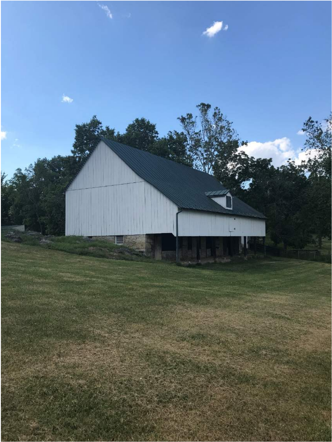
View to north west, showing east elevation and south gable elevation
