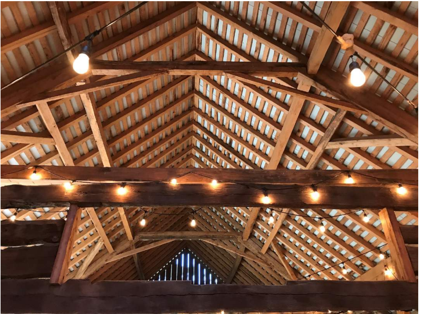
Detail of roofing structure
