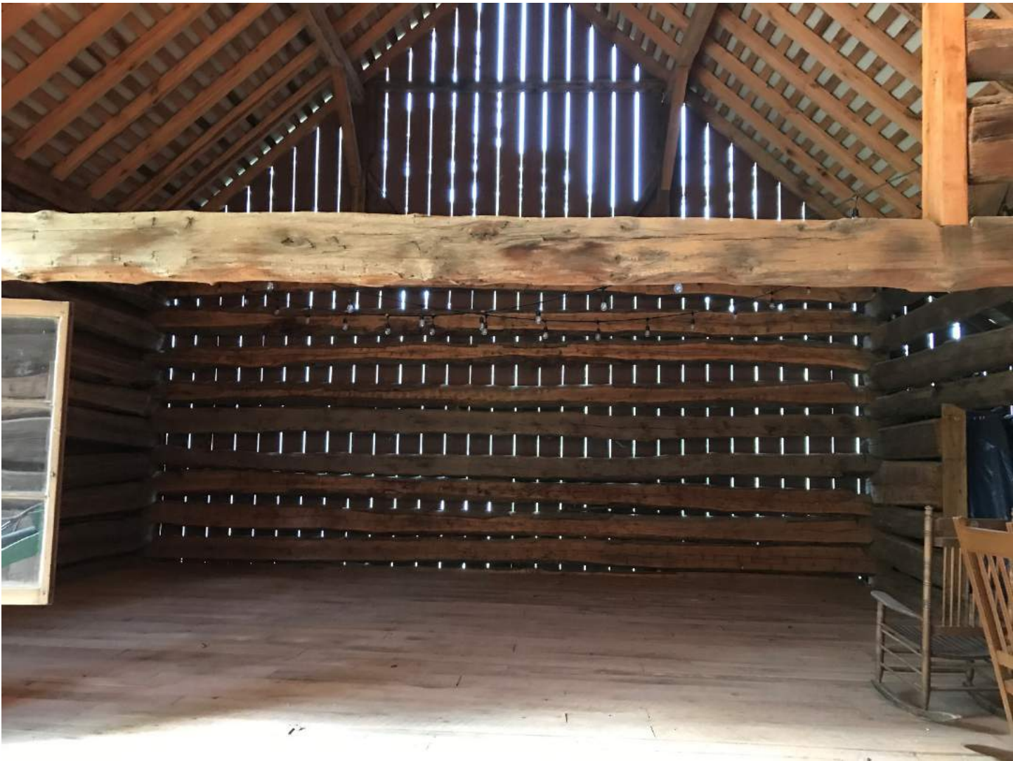
View to north gable, showing timber detailing
