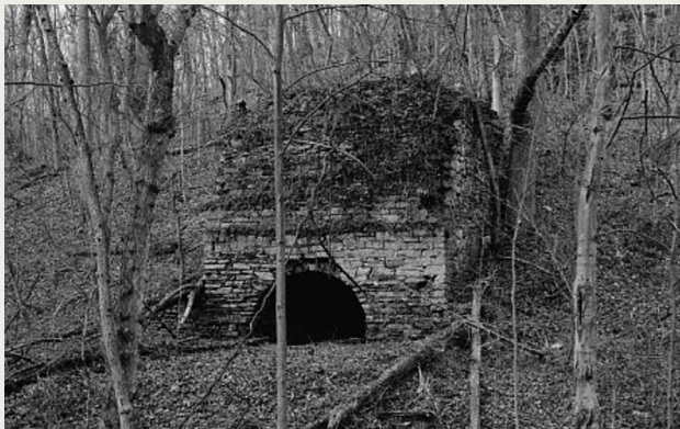
The first lime kiln at Boteler & Reynolds' cement mill, constructed in Shepherdstown in 1829. The natural cement produced there helped build the C&O Canal.
