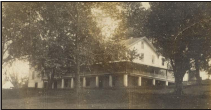
Figure 16. Shannondale Springs Hotel, uphill side, ca. 1913? Note the addition on the left side and the shed roofed addition visible on the right rear. Courtesy of the Jefferson County Museum.
