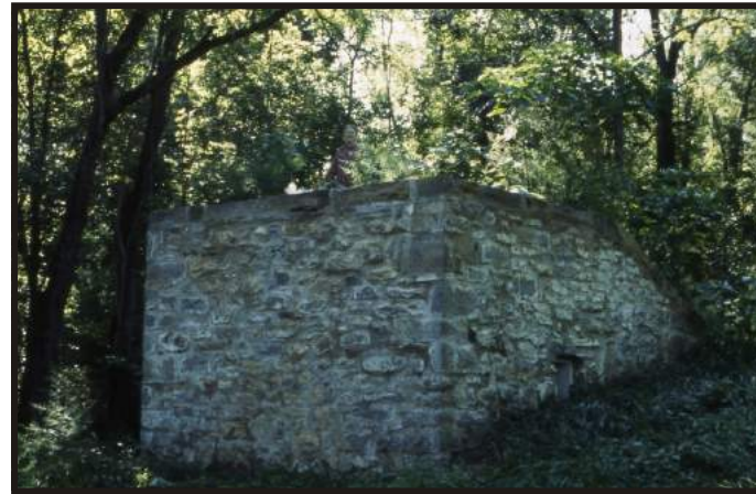
Figure 24. Shannondale Springs. Restored bath house, looking east. Summer 1997. Photographer, Carmen Creamer.
