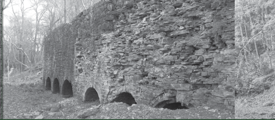
The battery of six kilns today, built 1829-1830. JEFFERSON COUNTY HISTORIC LANDMARKS COMMISSION, 2017.
