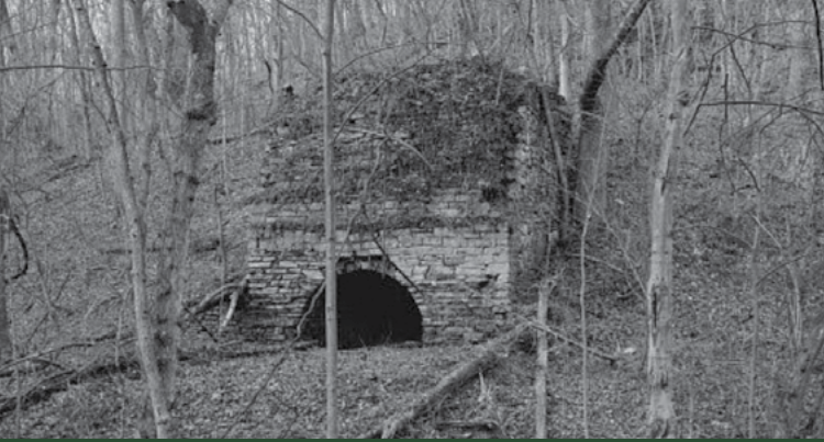
The first kiln, built 1828-1829. PHOTOGRAPHED FOR HAER WV-82, 1992. LIBRARY OF CONGRESS.
