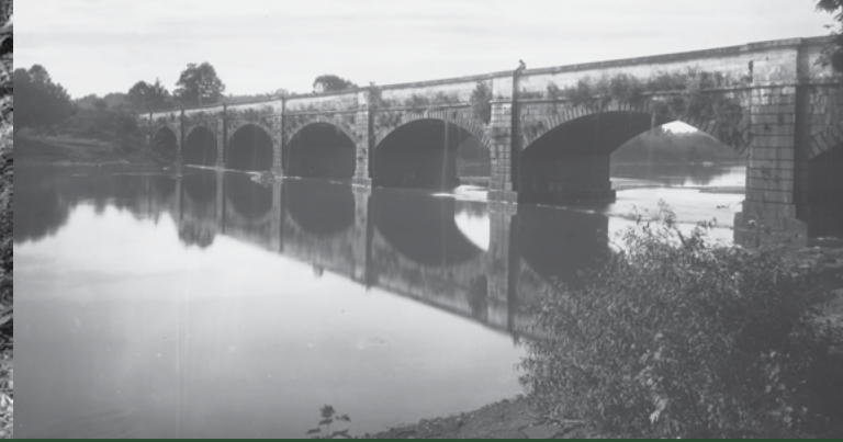
The Monocacy Aqueduct on the C&O Canal, built 1829-1833 with Shepherdstown cement and granite from nearby Sugarloaf Mountain. PHOTO C. 1892. LIBRARY OF CONGRESS.
