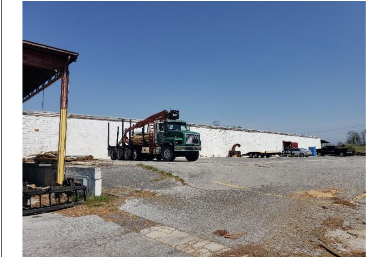
Image 7. Southwest side of the building, view toward the south corner.
