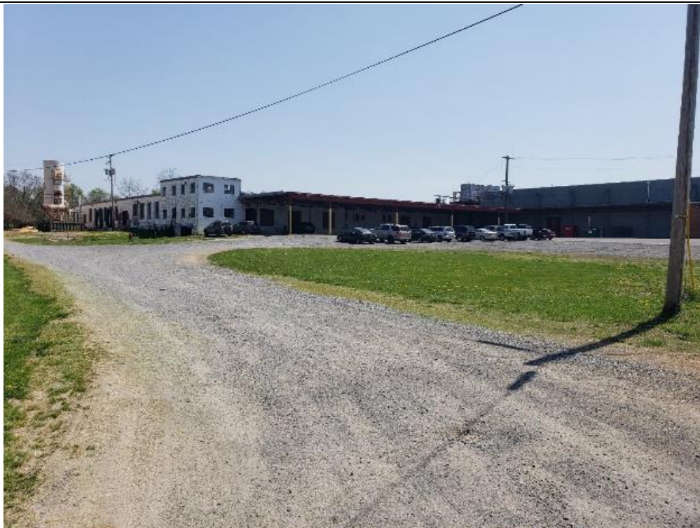
Image 4. Looking south toward the north corner of the building, with later addition visible on the right side of the photo.
