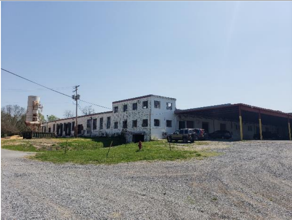
Image 3. Looking south, from the north corner of the building.
