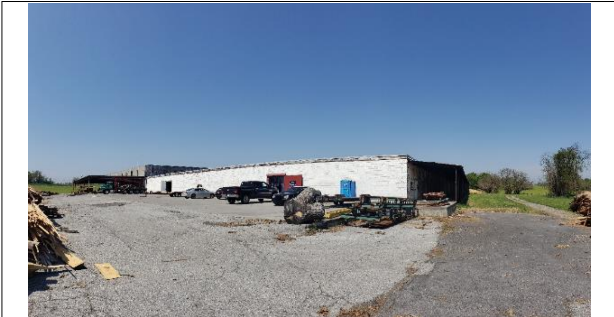
Image 8. Southwest side of the building, from the south corner.
