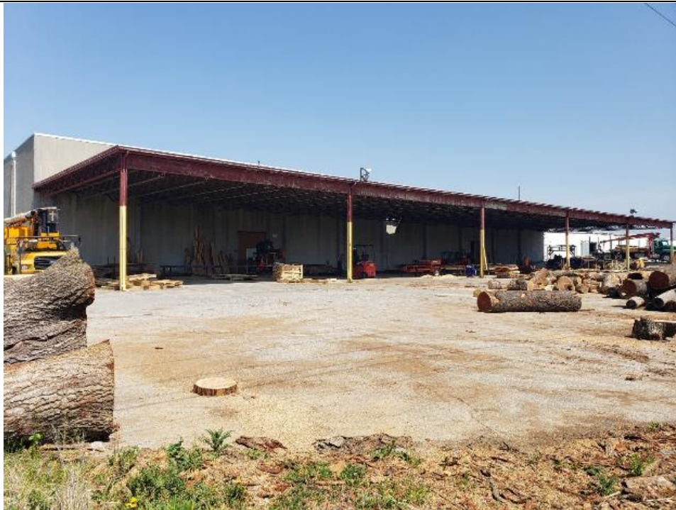
Image 6. West corner and southwest side of the building.
