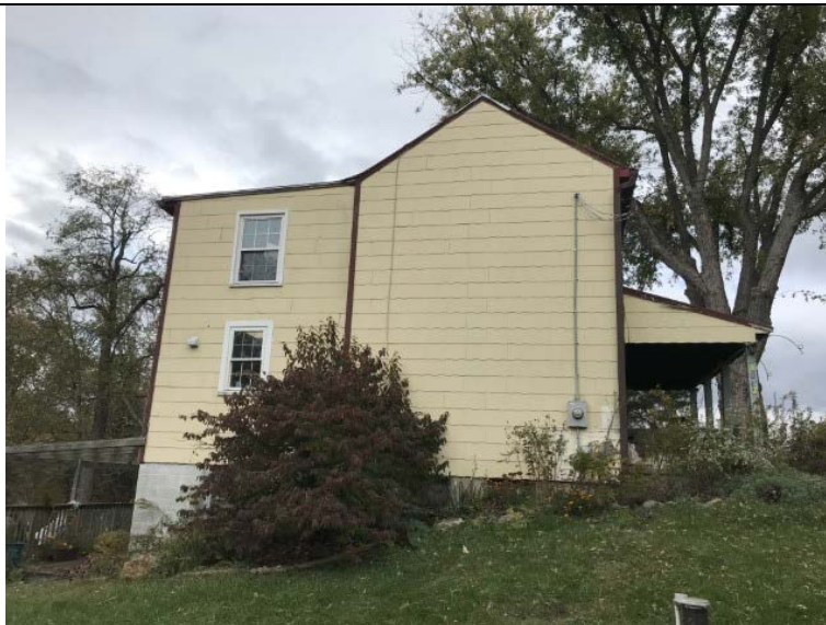
WV_Jefferson_County_Susan Thornton House_0002 Susan Thornton House east façade. View from east to west.
