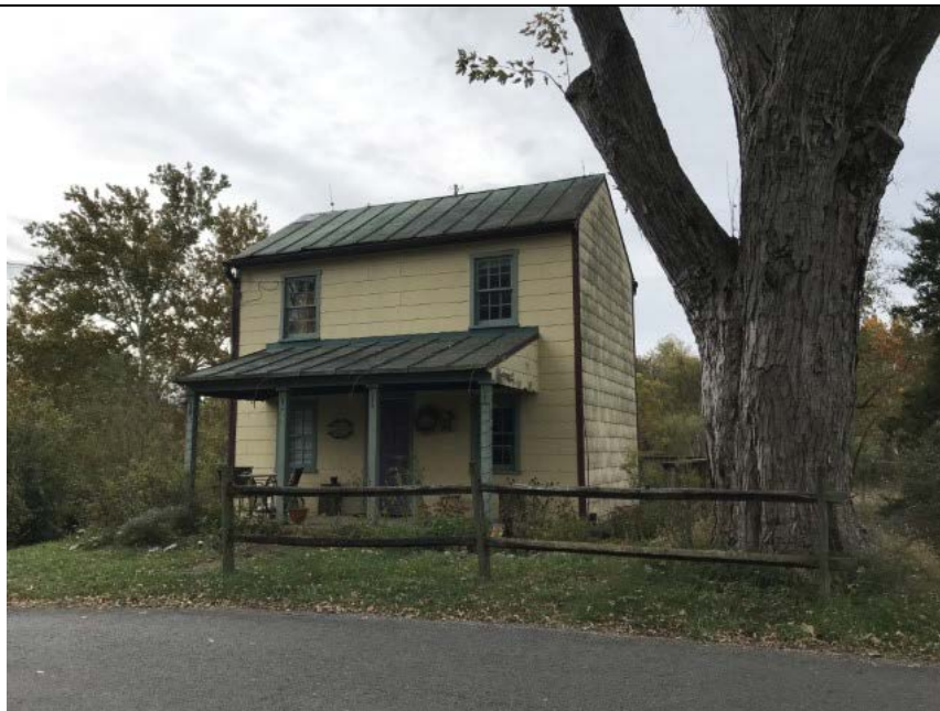
WV_Jefferson_County_Susan Thornton House_0006 Susan Thornton house. View northwest to southeast.
