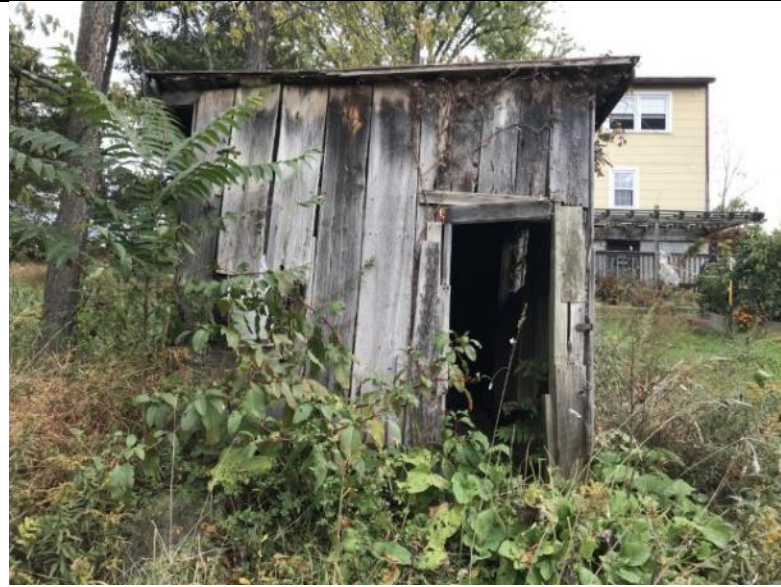
WV_Jefferson_County_Susan Thornton House_0009 Susan Thornton poultry house. View south to north.
