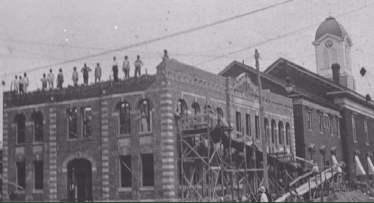
Photograph from 1918 showing the construction of the new jail behind the courthouse expansion. WV GEOEXPLORER.
